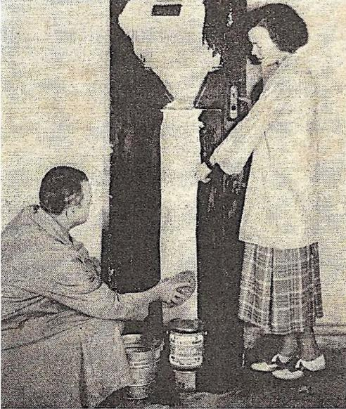
This new type of paint remover is applied with a brush, allowed to stand, and then wiped off with a sponge and water. No scraping is necessary, the remover doing all the work.
