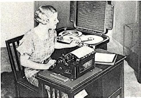
Using a magnet-sound process, this Magnetophon records sound on narrow bands of film which can be kept on file. Bands are inexpensive and resemble more costly talkie film.
