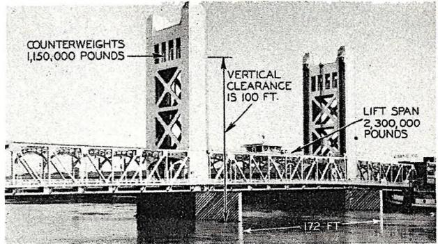
The new Tower Bridge across Sacramento River, in California, is the highest vertical lift span of any bridge in the world. It clears the river by 100 feet.
