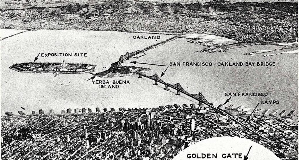
The San Francisco-Oakland Bay Bridge spans the largest navigable body of water yet bridged. No other bridge sweeps so high over the ships below. Over eight miles long, the west half of the bridge is in reality two suspension bridges.
